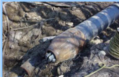
The D'Allesandro crew used a 14-inch diameter, reversible [Grundocrack](#) Koloss to replace 53 feet of 12-inch VCP storm sewer with 20-inch HDPE.
